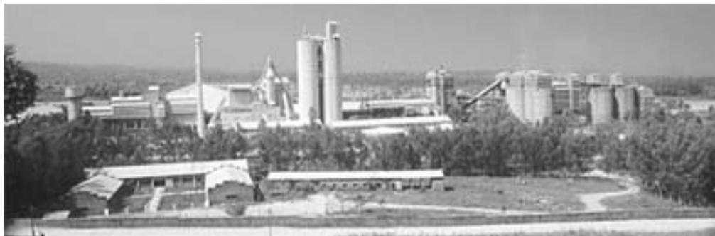
Cement is made by mixing chalk and clay and heating to very high temperatures in a coal-fired furnace. The coal forms soot and ash.
